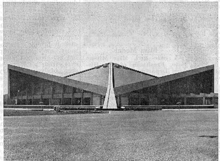
The Komazawa Gymnasium has adopted H.P. style, and the reinforced concrete building is surrounded by a sunken garden.
